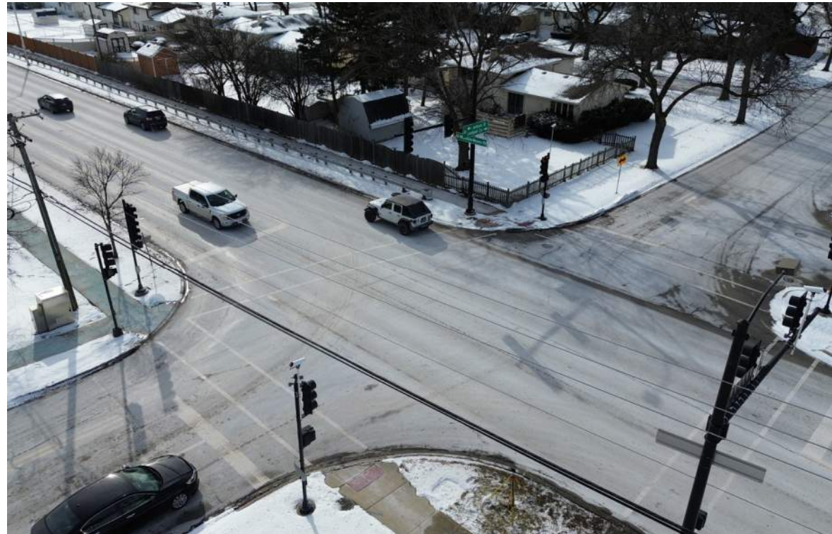
Westmore-Meyers Road at Jackson Street
