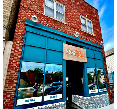
AWARDEE: NachoRita (14 W St Charles Rd) received a grant for new paint, repairing stonework, signage, and a commercial door.
