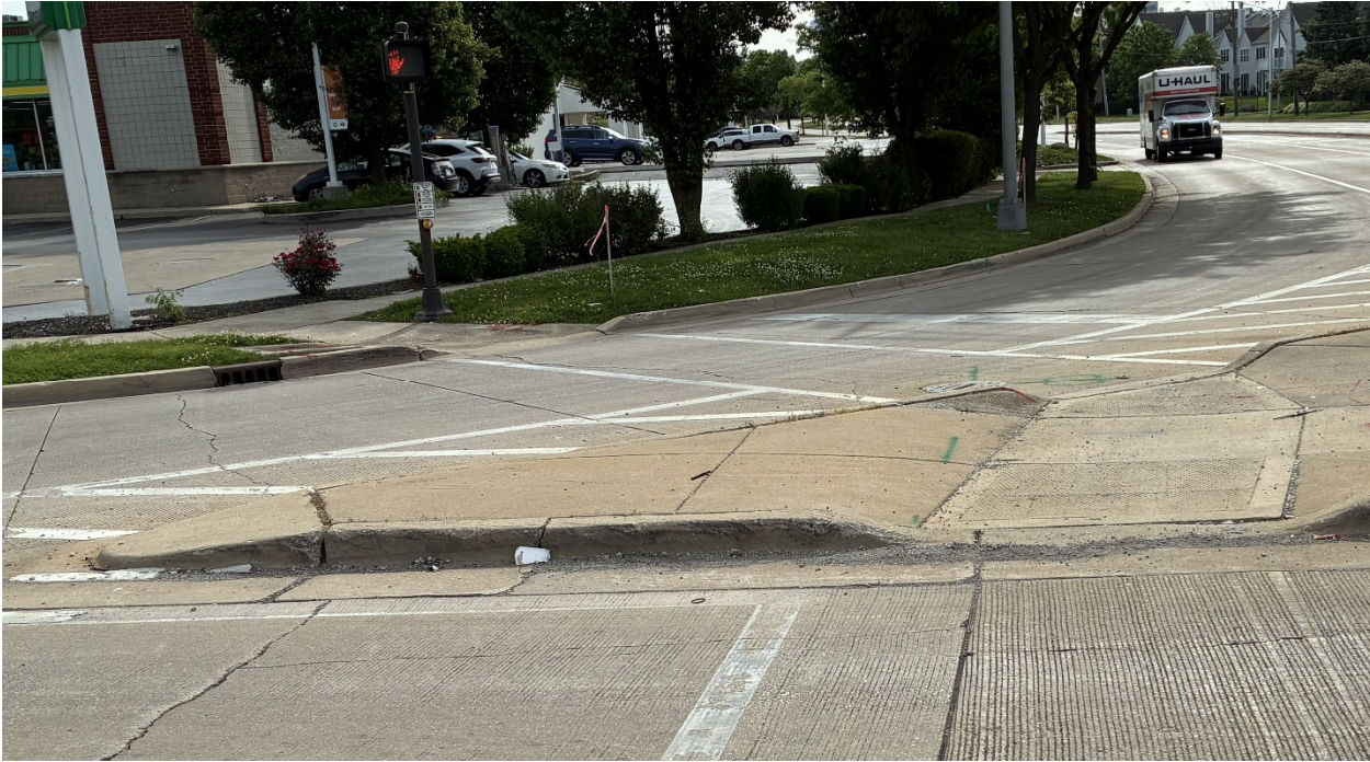
Photo #1 – Northbound Finley Road, just north of the intersection
