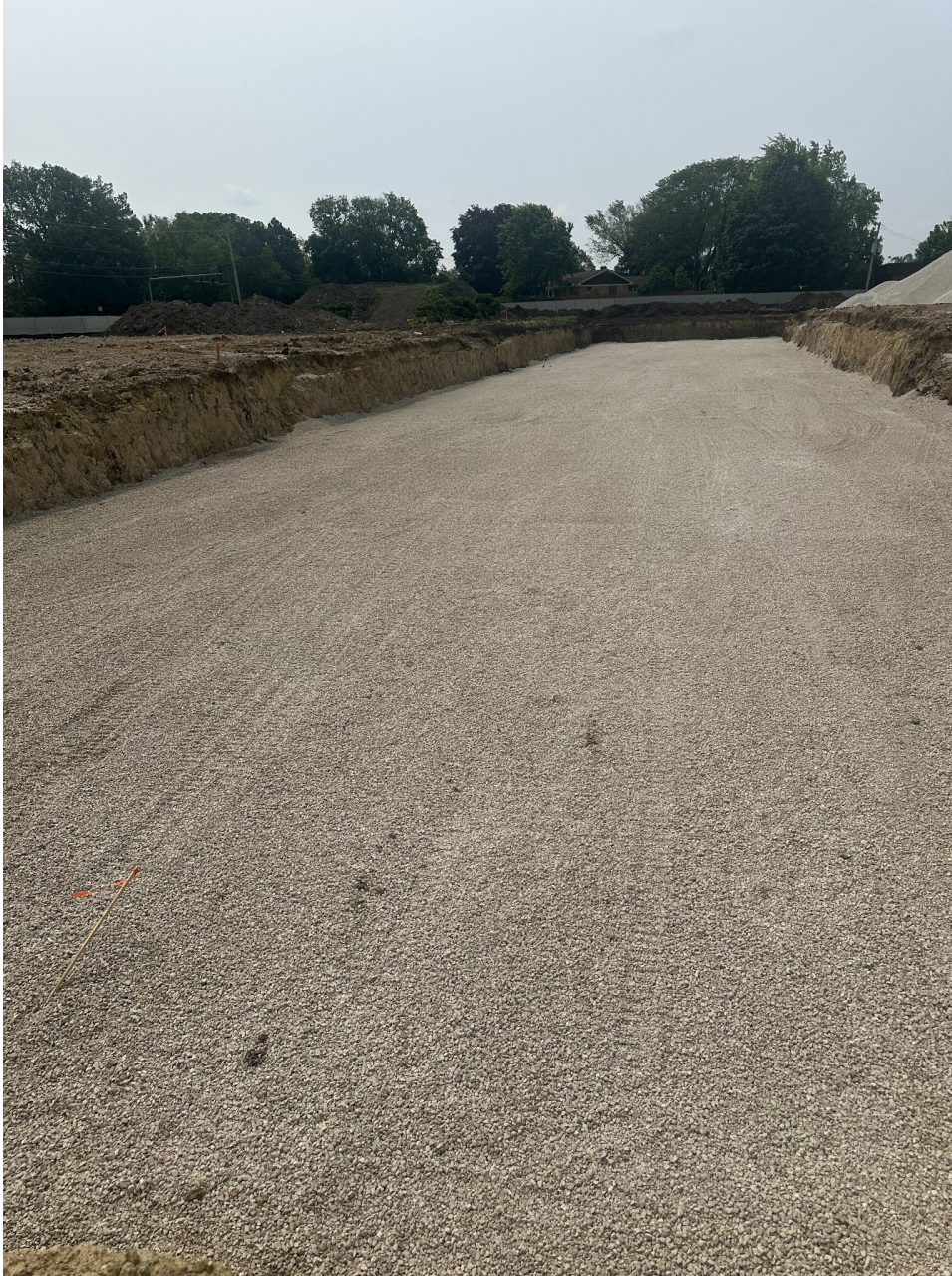
Figure 8: Detention Pit with Gravel Base – June 7, 2025
