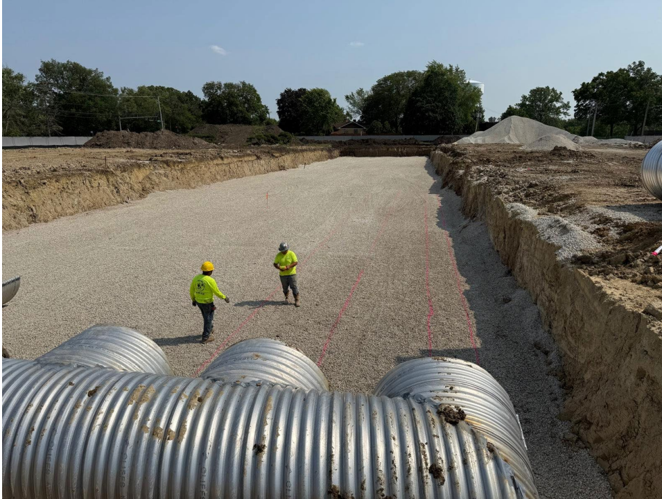
Figure 7: Detention Pipe Installation – June 10, 2025
