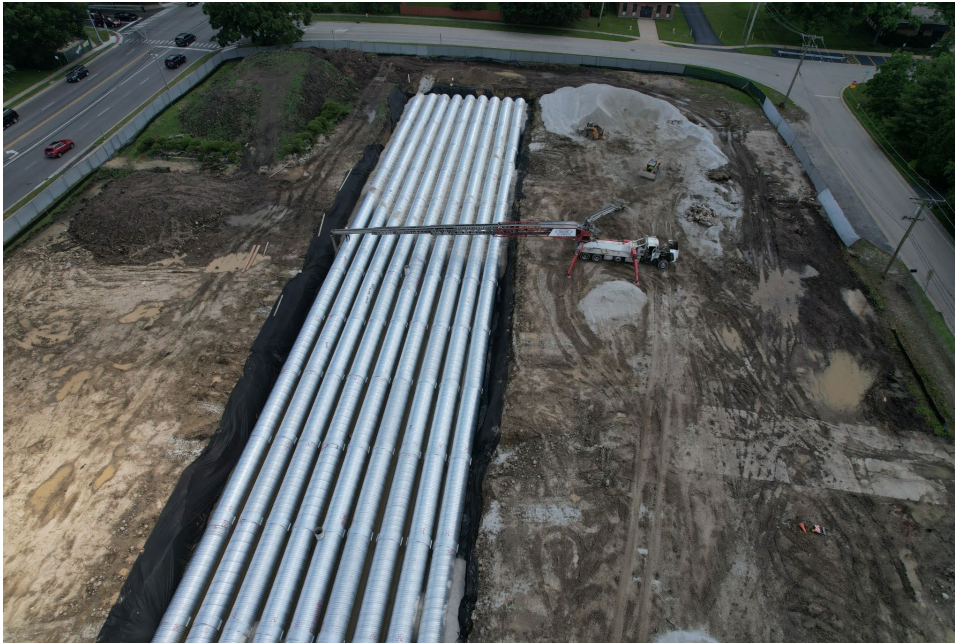
Figure 9: Aerial Drone View – June 19, 2025
