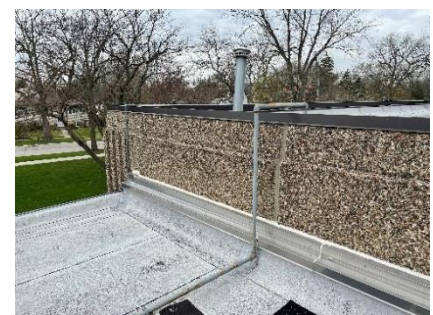
Repaired roof flashing
