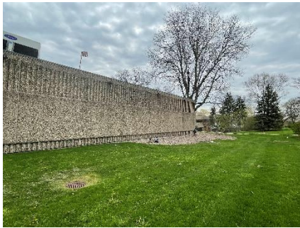
Exterior precast concrete wall
