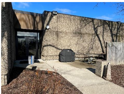
Existing exterior light fixtures
