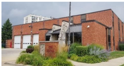
Lombard Fire Station 45
