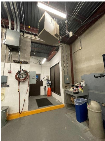
Sally Port / Garage structure
