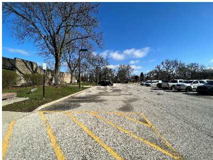
Shared parking lot for staff and visitors
