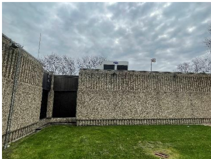
Exterior precast concrete wall
