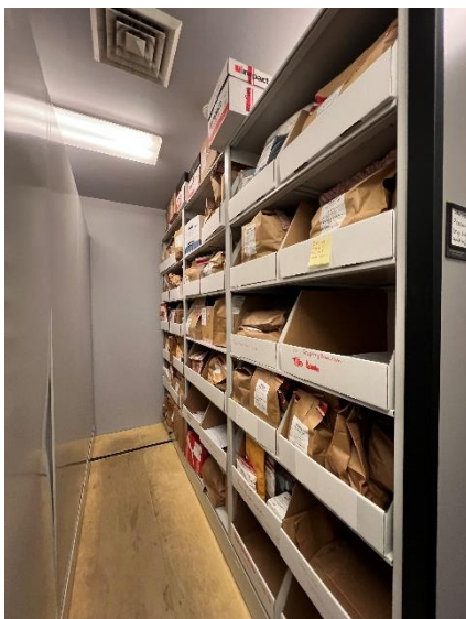
Insufficient ventilation in Evidence Storage room
