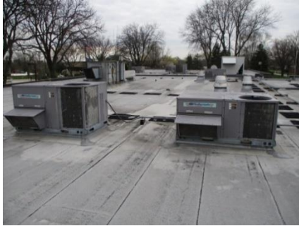
Existing rooftop units
