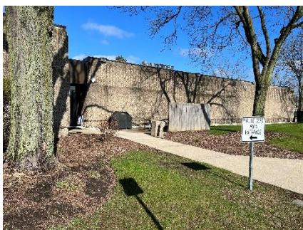
Staff entrance is not secure
