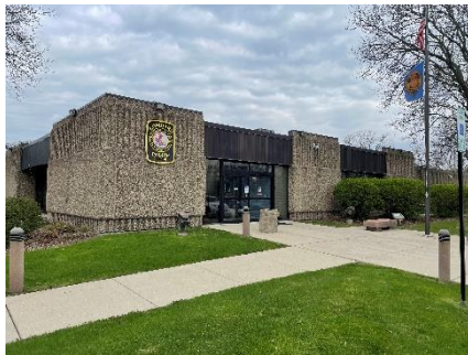
Main entry of police station
