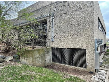
Existing grade at Village Hall
