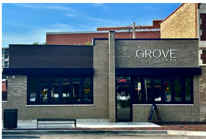
AWARDEE: Grove Tavern (2-8 W St Charles Rd) received a grant for the full build out of this new restaurant. The property at 8 W St Charles Rd was previously a vacant lot.
