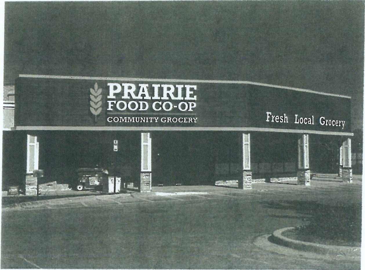
Photograph of Erected Channel Letter Wall Signage
