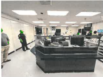
Booking room – note steel cell construction to left which do not allow sound separation
