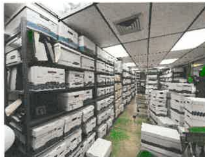
File boxes stored too close to ceiling
