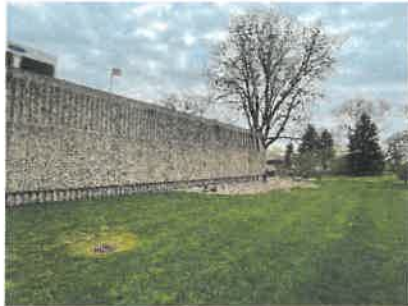
Exterior precast concrete wall
