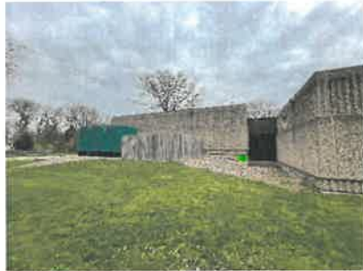
West elevation of Apparatus Bay
