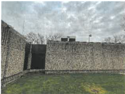
Exterior precast concrete wall
