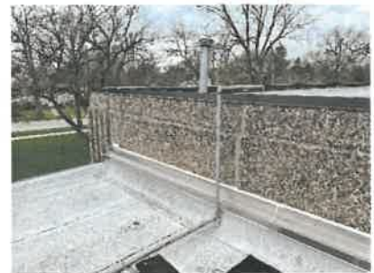
Repaired roof flashing
