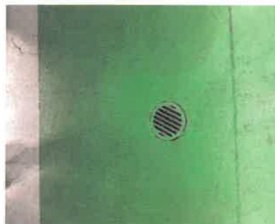
Floor drain in Firing Range
