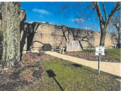
Staff entrance is not secure
