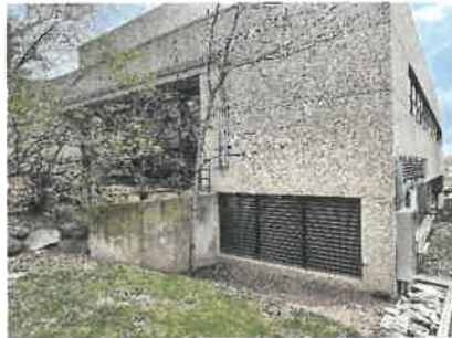
Existing grade at Village Hall
