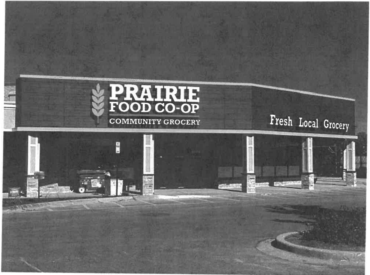
Photograph of Erected Channel Letter Wall Signage
