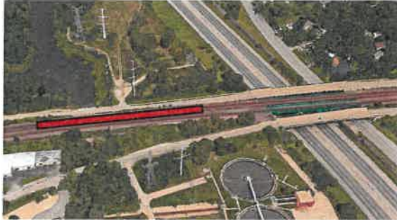
Aerial view of Crescent Boulevard, west of I-355 (wall location highlighted)
