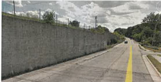
Crescent Road looking southeast
